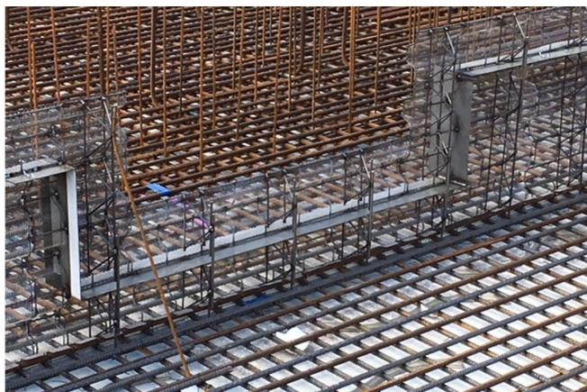
Formwork elements for working joints Stremaform® with coated metall waterstopp
