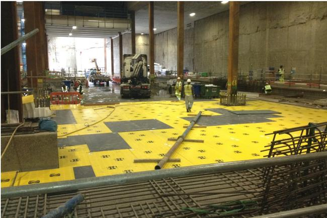
Pecavoid® installation at Heathrow T2B
