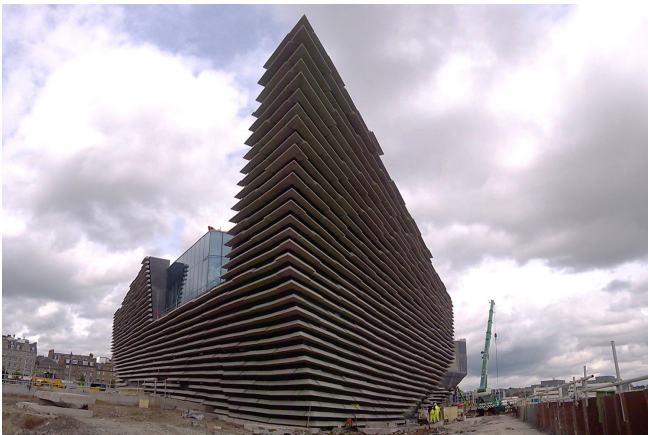
V&A precast cladding in position © www.maxfrank.com
