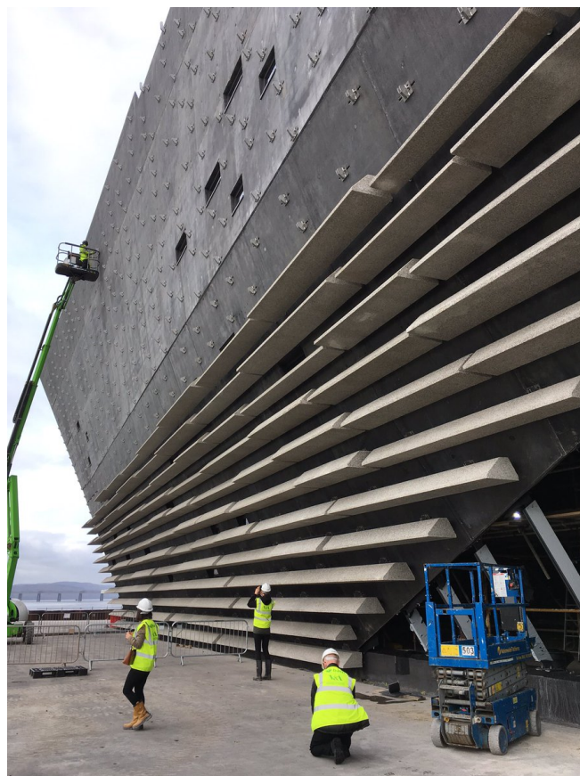
V&A Zemdrain® concrete finish and cladding © www.maxfrank.com
