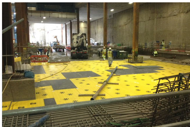
Pecavoid® installation at Heathrow T2B © www.maxfrank.com
