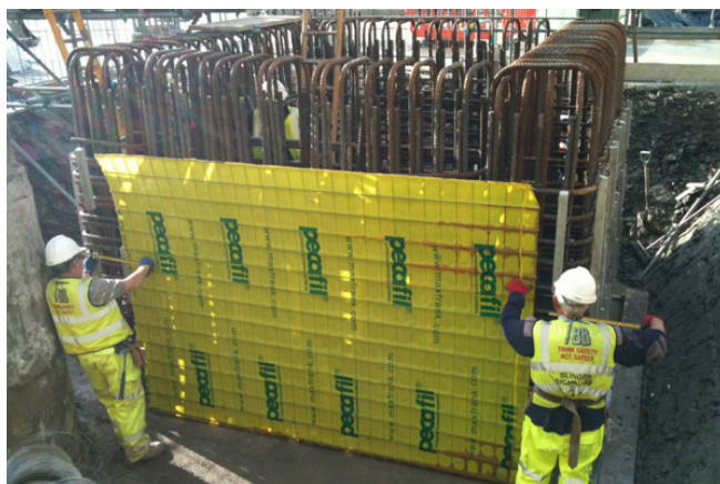
Pecafile® installation at Heathrow T2B © www.maxfrank.com
