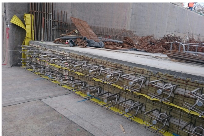
Formwork element with integrated shear force dowels © www.maxfrank.com
