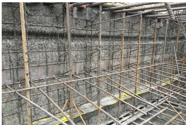
Stremaform® formwork elements for working joints © www.maxfrank.com
