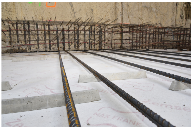
Fibre concrete bar spacer between sub-structure membrane and reinforcement
