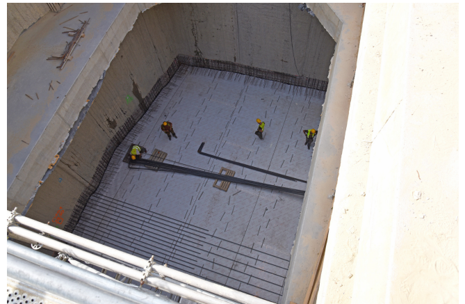
Start of reinforcement laying on surface spacers © www.maxfrank.com
