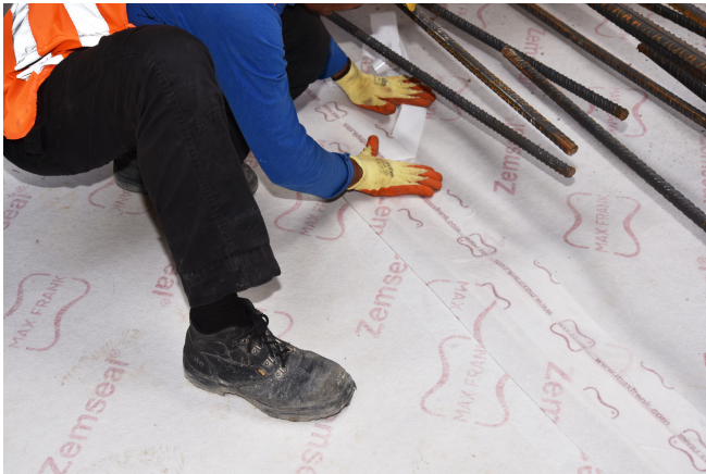
Simple butt joint formation of Zemseal® membranes © www.maxfrank.com
