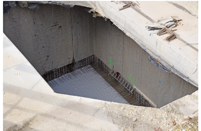
Shaft chamber with laid Zemseal® waterproofing membrane © www.maxfrank.com
