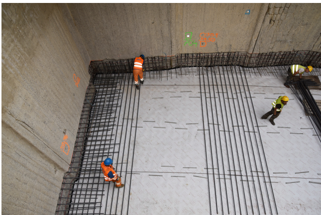
Laying the lower reinforcement layer © www.maxfrank.com
