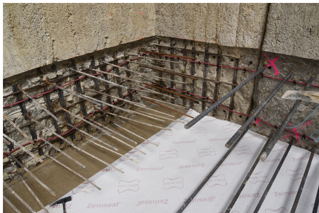
Sealing of the highly reinforced connection area with two grouting circuits of Intec® Premium injection hose
