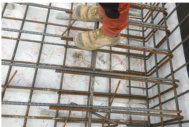
Zemseal® waterproofing membrane installed © www.maxfrank.com
