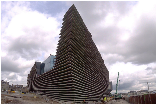
V&A precast cladding in position © www.maxfrank.com
