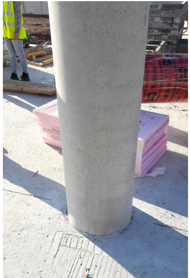
Column formers Tubbox® - blowhole free finish © Krešimir Caharija, www.possum.hr
