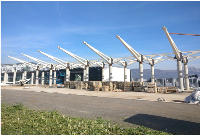
Column formers Tubbox® - blowhole free finish © Krešimir Caharija, www.possum.hr
